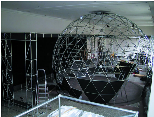
Figure 8: The dome during installation
